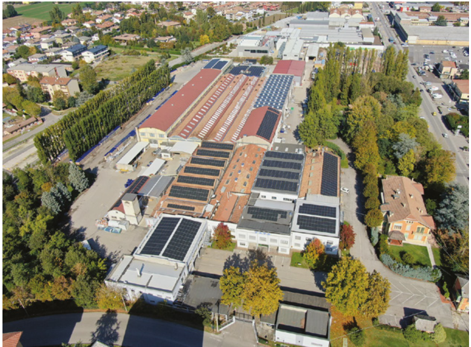
Aerial view of Fava facilities.
